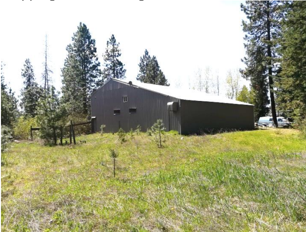
Shipping and receiving structure north of Hern Avenue west of lot 4 (Building B2)
