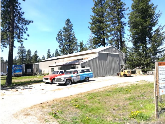
Metal fabrication and storage building north of Hern Avenue nearest to Atlas Road (Building B6)
